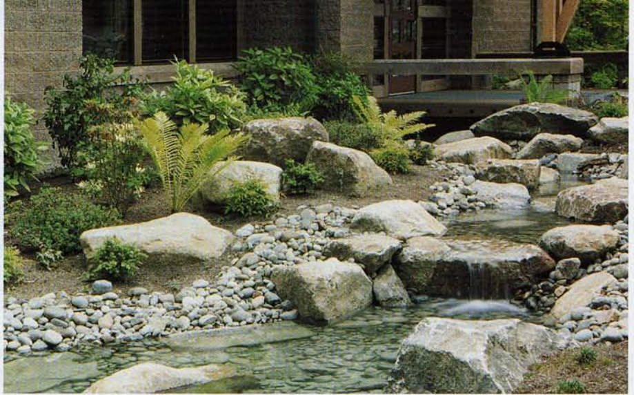
The stream, above and left, receives stormwater from the building's roof. Any overflow goes to a biofiltration swale, shown below.
